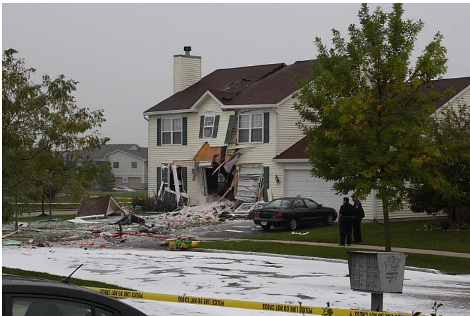
Smashing out the front door area
