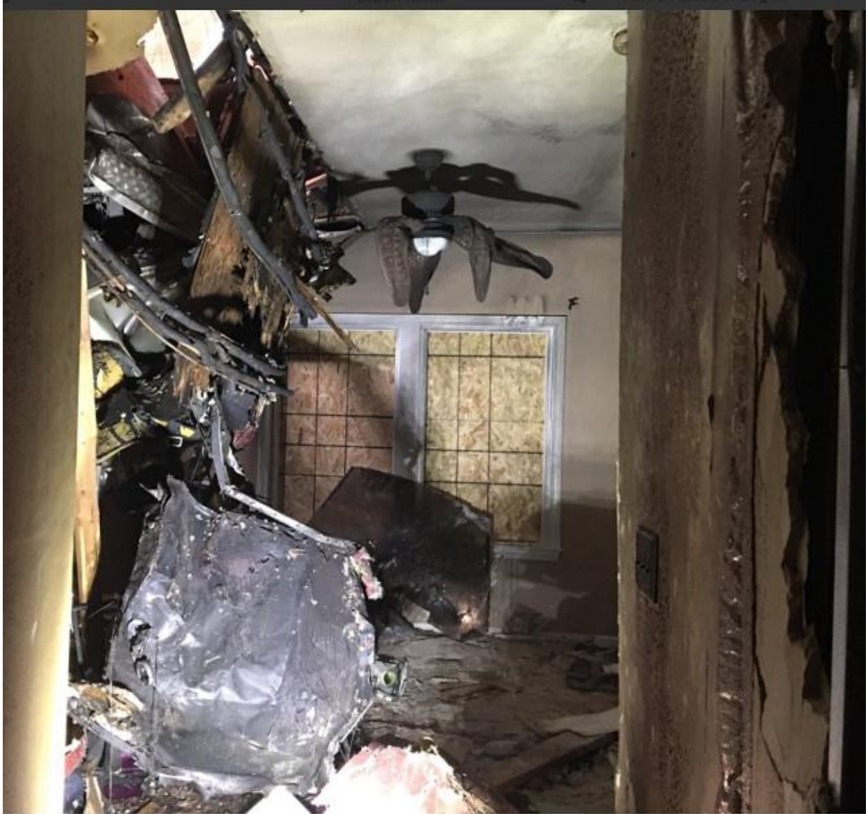
Burned interior of condo showing Experimental Amateur Built (E-AB) airplane crash impact
